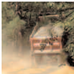
Dump trucks hauled in many loads of gravel and rock to repair and stabilize the White Pines Trail.
